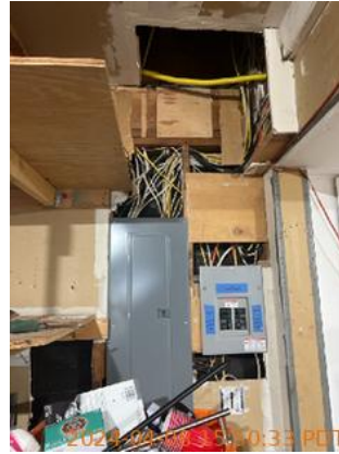
Electrical/Exposed Wiring
