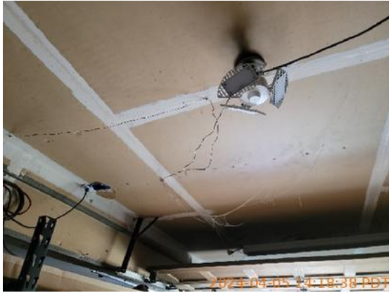
Electrical/Exposed Wiring
